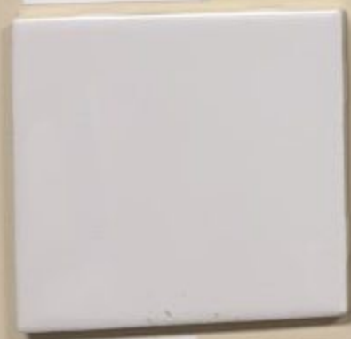
Restroom Walls Field Tile Daltile D100 White
